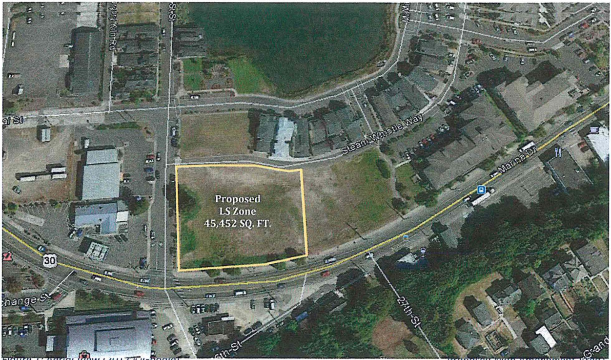
Figure 1: Aerial View (2017 ©Google)
